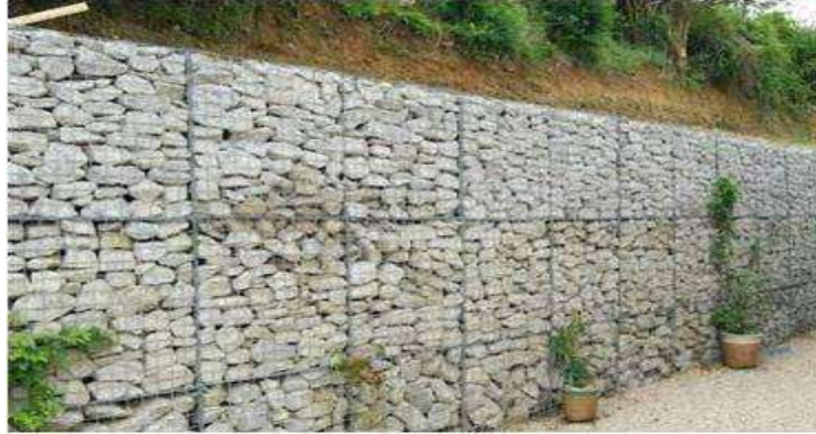
Fig 12:- Gabion masonry
