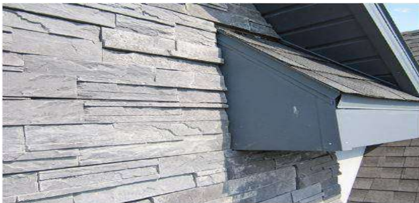
Fig 11:- Veneer masonry
