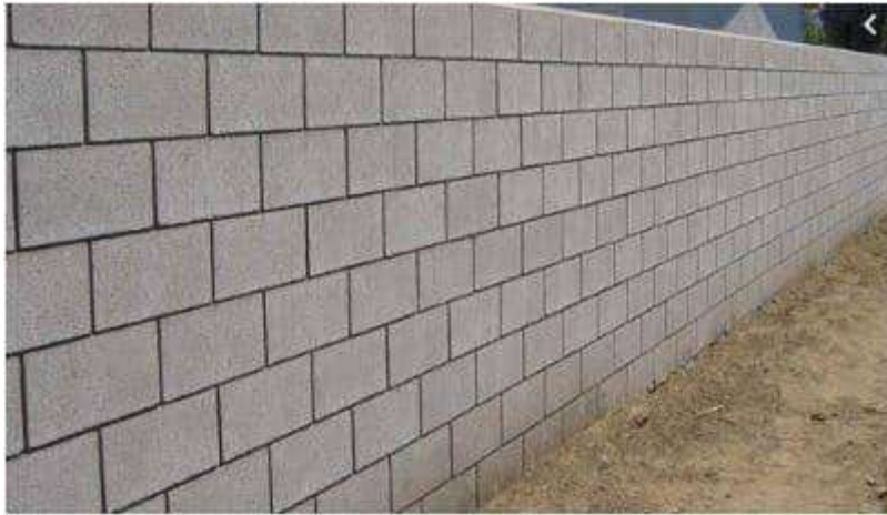
Fig10:- Concrete block masonry
