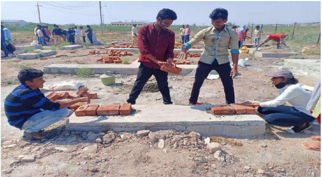
Plate 4&5:- Construction of masonry wall
